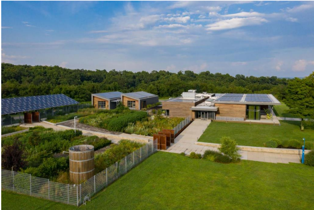
Figure 2: Aerial view of solar PV panels installed at Eden Hall Campus, Chatham University
