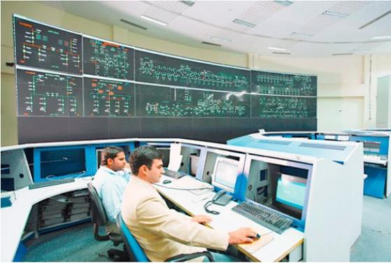
DMRC’s SCADA system tracks and monitors all interruptions, including seconds of voltage fluctuation causing momentary interruptions. The entire energy infrastructure is designed to prevent flooding of underground stations, sub stations and diesel generation systems. Strategies and design considerations were implemented to prevent damage from wind storms and seismic activities.
