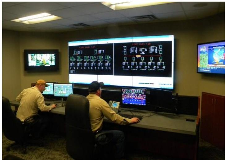
In addition to the SCADA system, Fort Knox has installed smart meters enabled with bidirectional communication between the facility and the utility. The control center transforms data generated by these smart meters into a detailed, 3D optical energy report which provides a visualization of building energy data that can be used to better manage the whole facility for sustained results.
