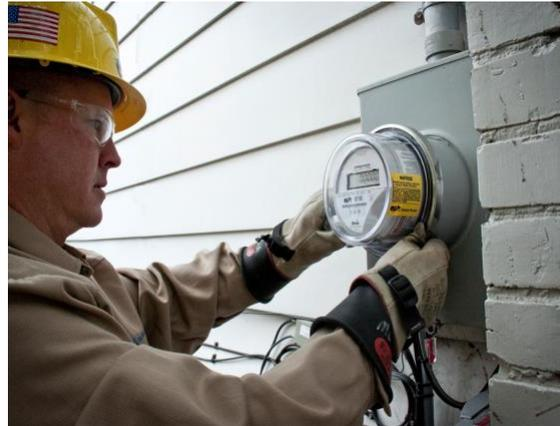
*Figure 3: Installation of Smart Meters by EPB personnel for homes*
