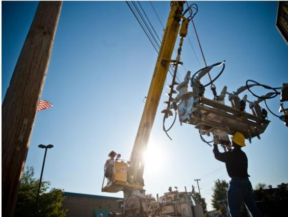
*Figure 2: Installation of Smart Switches across EPB distribution network*
