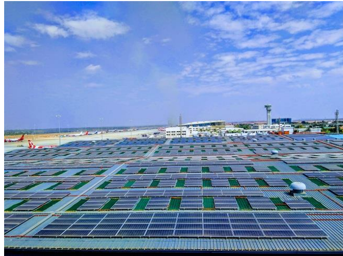
Figure 2: BIAL - Onsite rooftop solar PV system
